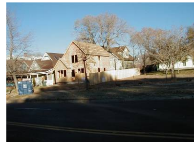
New house under construction. (Photo courtesy of Utah State Historic Preservation Office.)
