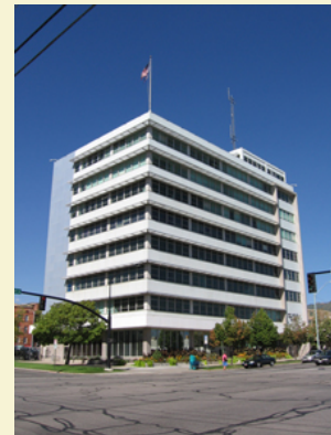
Salt Lake City Public Safety Building (Historic Northwest Pipeline Company Headquarters), 1958, is an example of a significant modern resource that has just recently reached the 50-year milestone.
