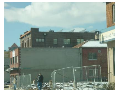
(top) Solar panels in a west side neighborhood. Additional design guidelines could help minimize the profile of such panels in historic districts.
